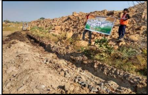
Cleaning of Garland drain & strengthening of Bunds along the waste dump
